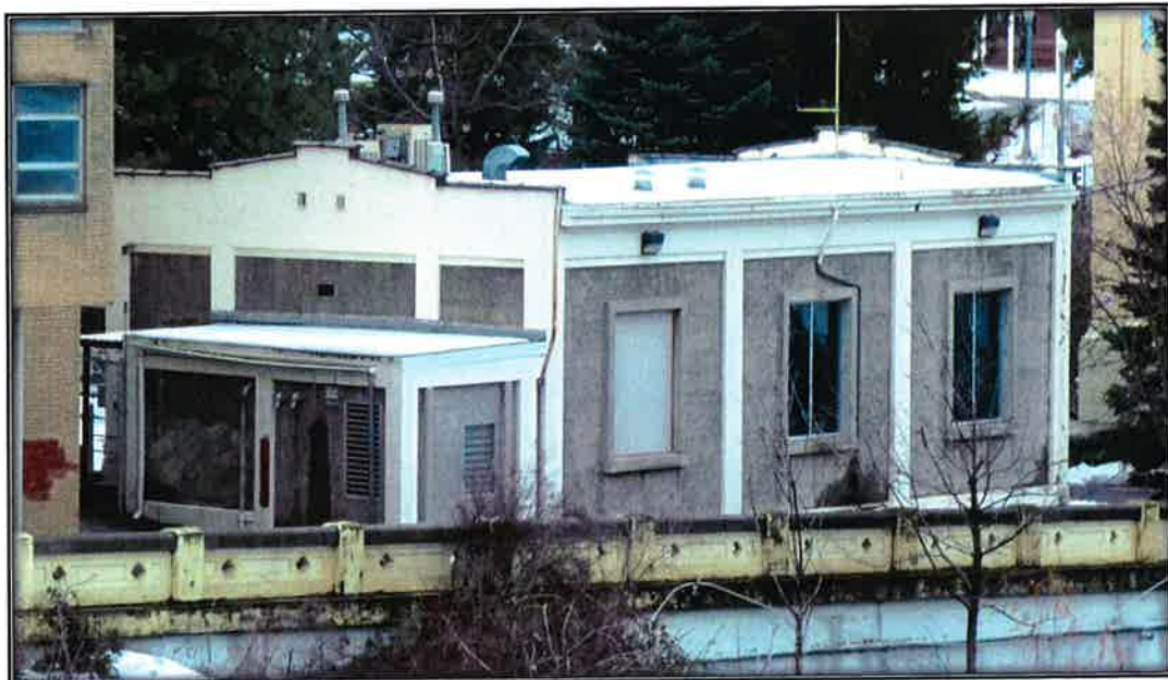
Figure 6: Southwesterly view toward the building and the rooftop.
