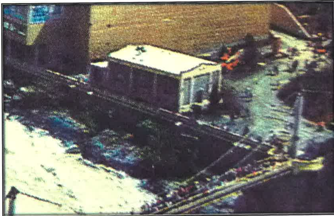
Figure 9: Southeasterly aerial image of the building revealing windows and east end addition, 1974 (Northwest Room).
