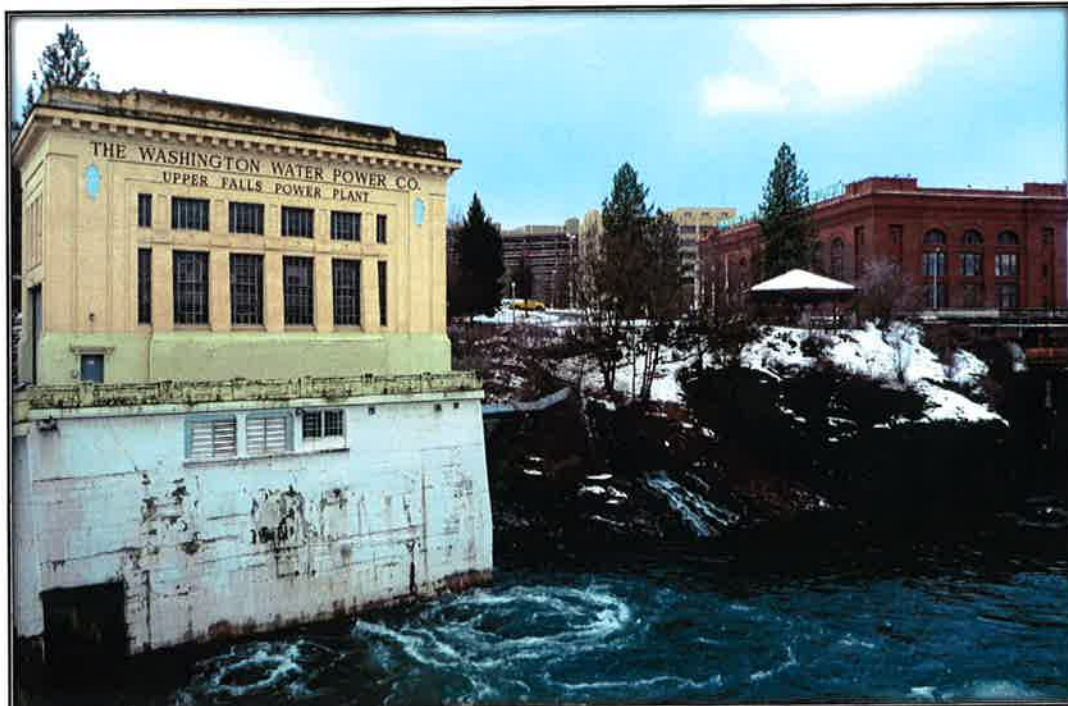
Figure 2: Southwesterly view toward the Upper Falls and Monroe Street Powerhouses and a portion of the concrete railing.
