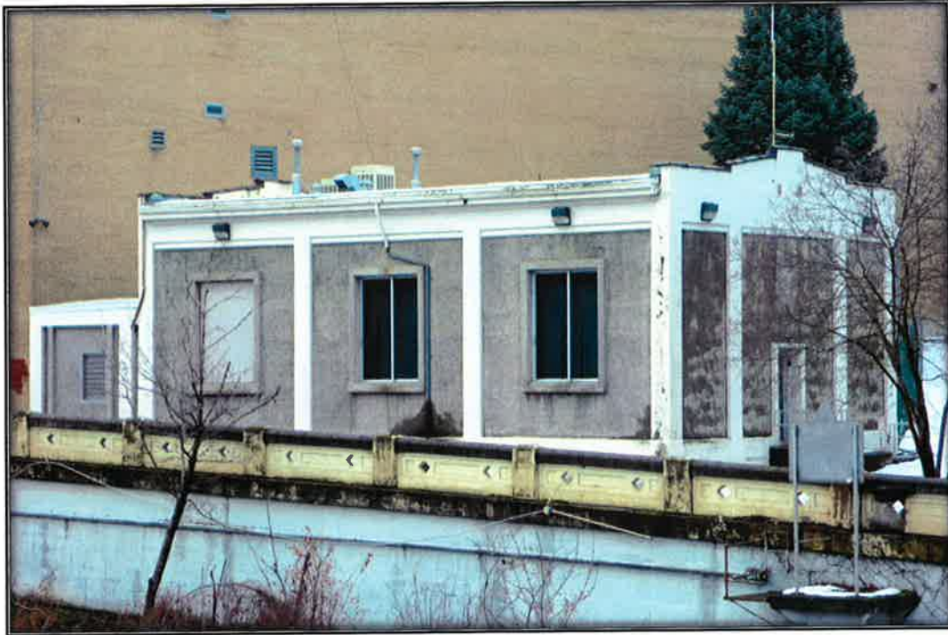
Figure 1: Northwest corner of the Old Fire Dispatch Building.
