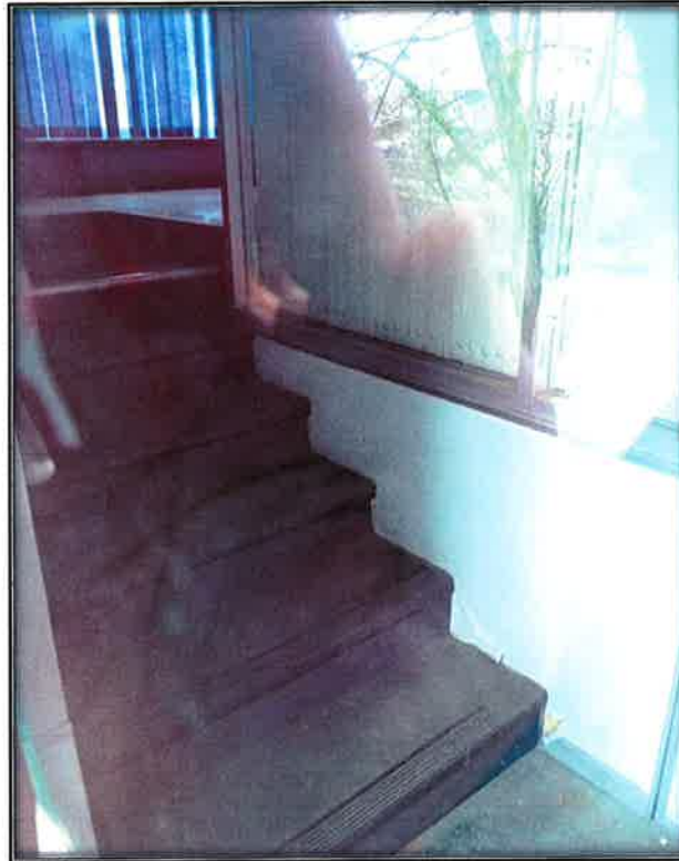
Figure 15: View toward the interior and raised floor from front door.
