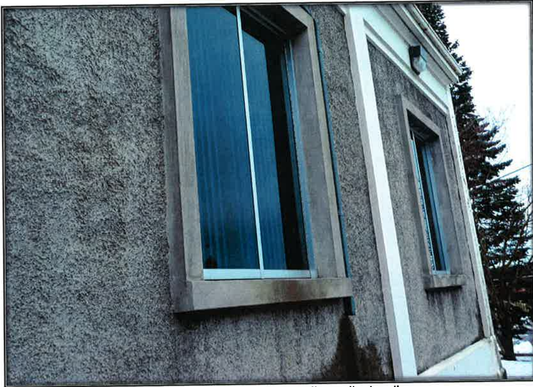
Figure 13: Nonhistoric windows on the north elevation.
