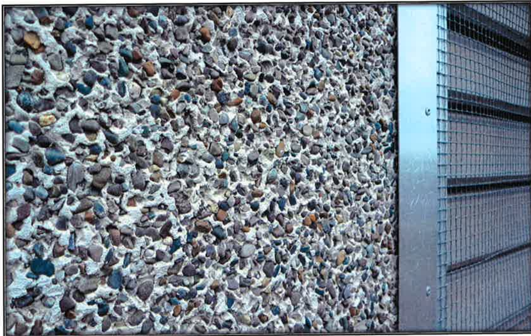
Figure 12: Aggregate finish on east addition.
