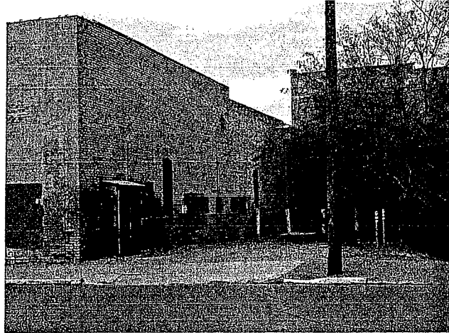
EAST EXTERIOR SIDE OF BUILDING
