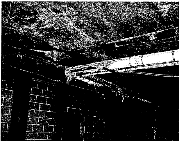
VIEW OF DETERIORATED ACM-TSI PIPING INSULATION IN SOUTH HALF OF BASEMENT
