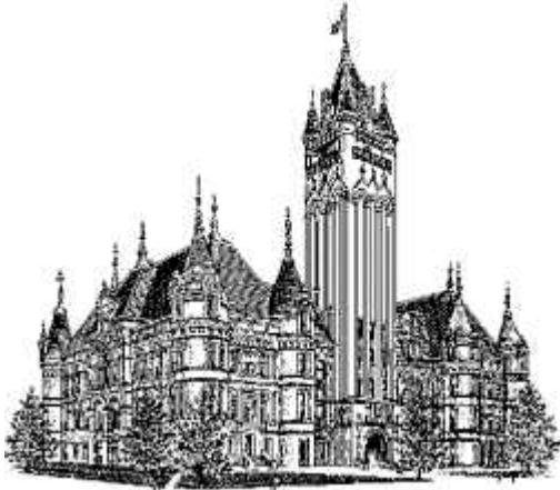
SPOKANE COUNTY COURT HOUSE
