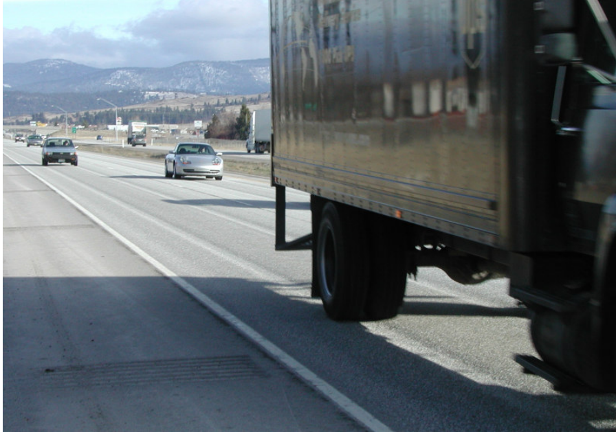
Photo 14. Wear due to studded tires on a hot mix asphalt pavement (I-90 in the vicinity of the Idaho Border).
