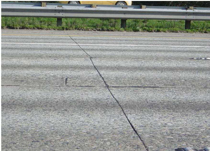
Photo 10. Concrete pavement on I-5 near Boeing Field. ADT: 204,000 vehicles Pavement Age: 34 years
