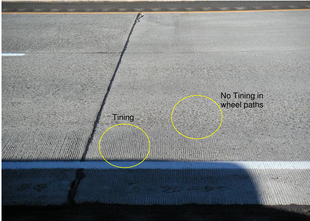
Photo 3. Concrete pavement on SR-395 south of I-90. ADT: 6,800 vehicles Pavement age: Eight years
