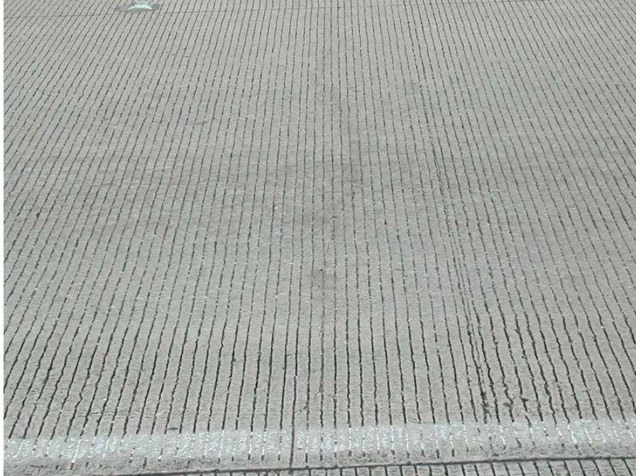
Photo 5. Concrete pavement on I-45 in Houston, TX. ADT: 178,000 vehicles Pavement Age: 16 years
