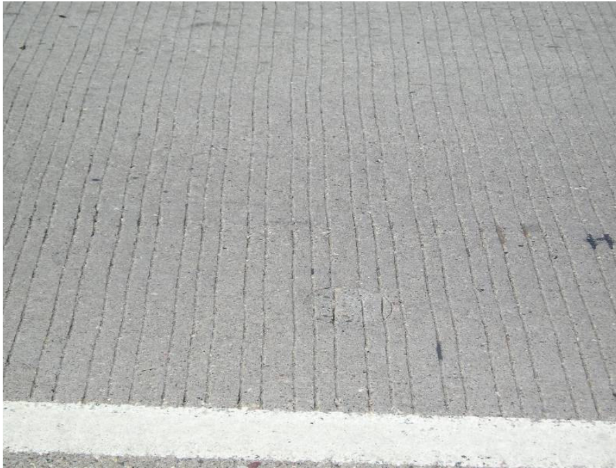
Photo 7. Concrete pavement on I-94 in Minneapolis, MN. ADT: 130,000 vehicles Pavement Age: 28 years
