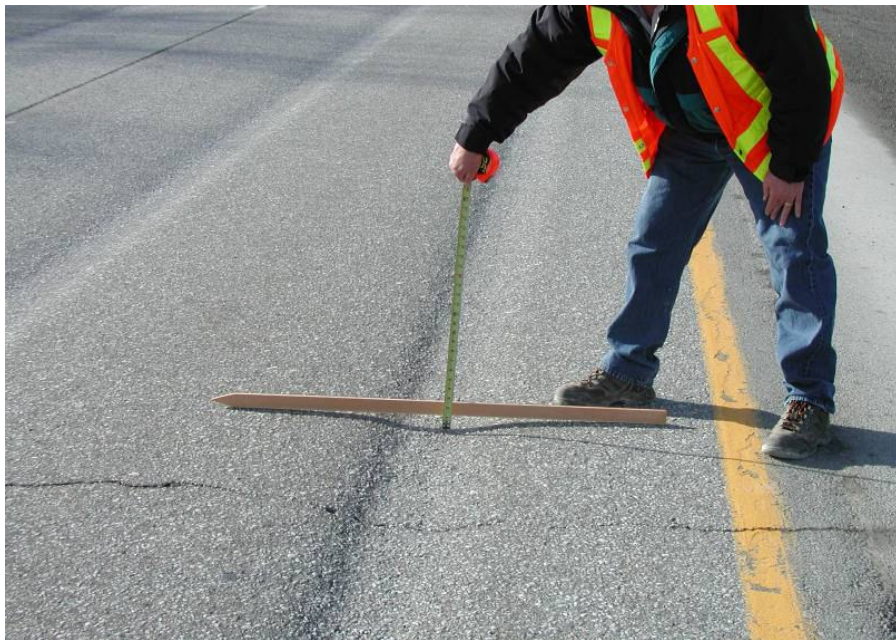
Photo 15. Studded tires raveling on hot mix asphalt pavement on I-90 vicinity of Idaho border.
