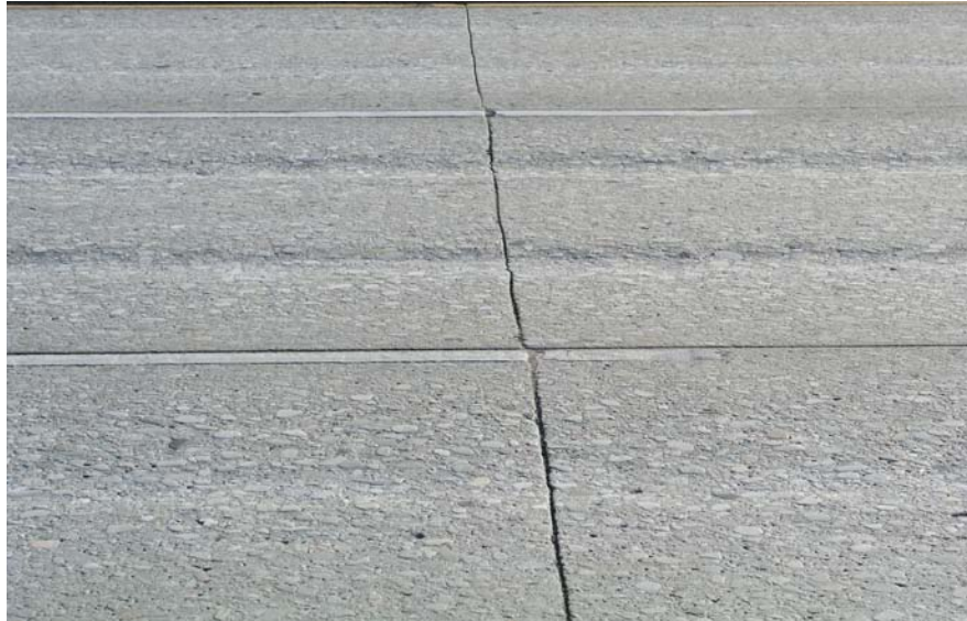
Photo 12. Concrete pavement on I-90 in Spokane. ADT: 100,000 vehicles Pavement Age: 48 years
