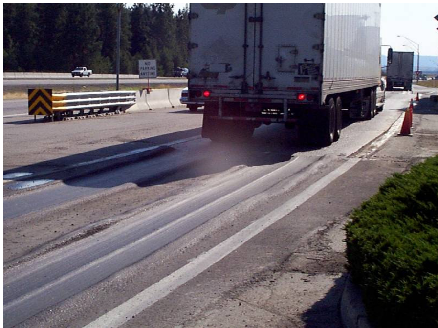
Photo 13. Spectacular, but not typical, hot mix asphalt pavement rutting (I-90 Port of Entry Weigh Scale, Spokane vicinity).
