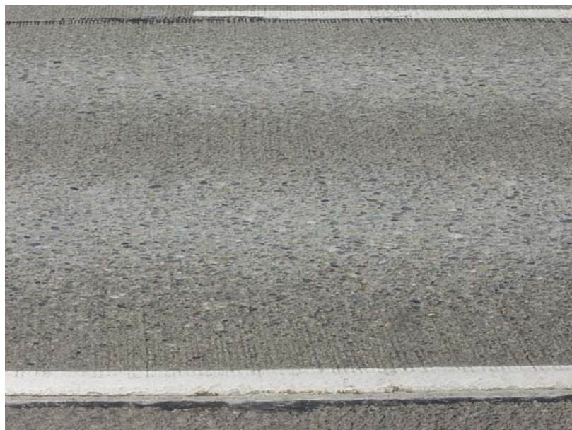
Photo 8. Concrete pavement on I-90 near Preston Fall City. ADT: 50,000 vehicles Pavement Age: 28 years
