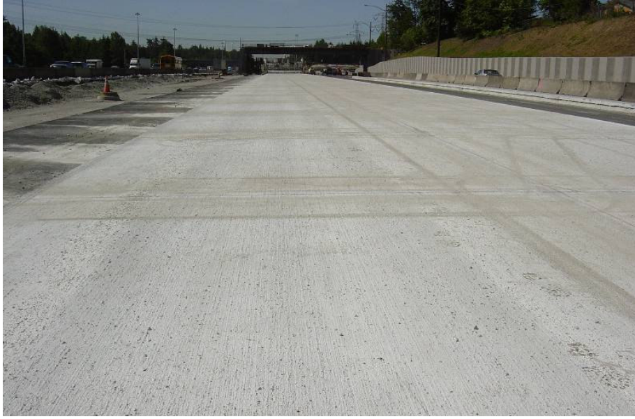
Photo 1. New concrete pavement on southbound I-5 in the vicinity of 317 th Constructed 2005, not yet under traffic.
