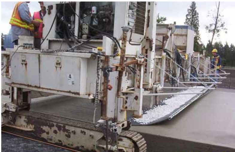
Photo 2. Texturing concrete pavement with an Astroturf Drag
