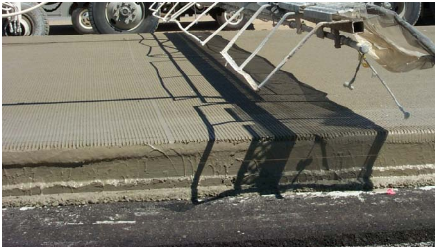
Photo 4. Transverse tining of fresh concrete pavement.
