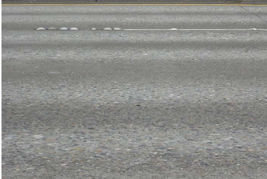
Photo 11. Concrete pavement on I-5 near the Tacoma Dome. ADT: 194,000 vehicles Pavement Age: 40 years
