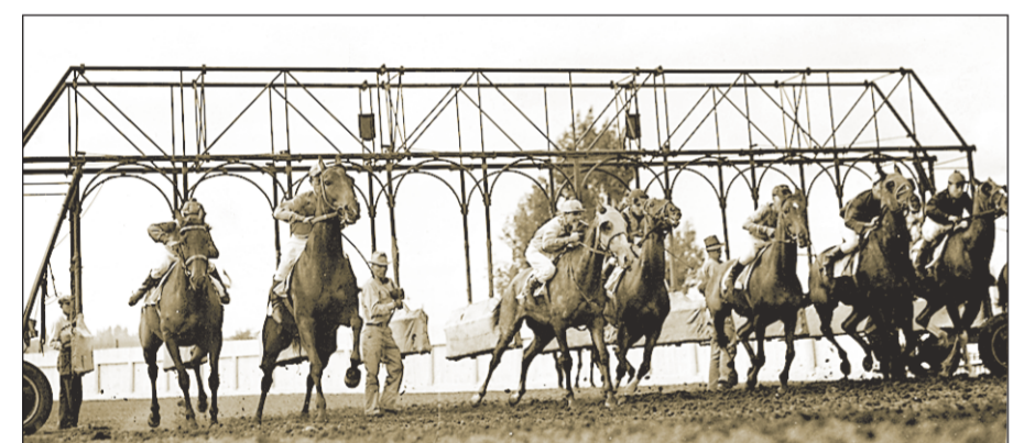
There they go in 1937: Starting-gate pioneer Clay Puett designed and built this open-stall gate for his use as the starter during Playfair's first few seasons.
