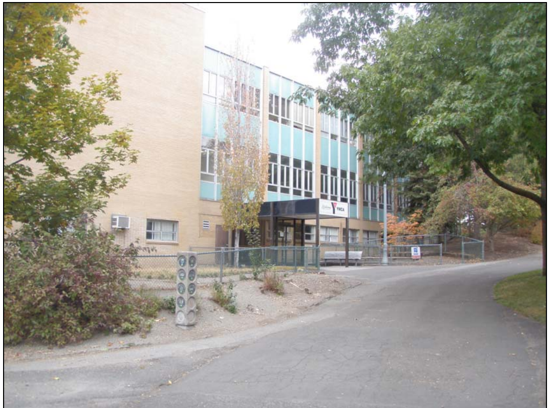
4. The subject's south elevation, facing northeast. The main entry to the former YMCA is shown, which leads into the first floor (also known as Basement 1 of three basement levels).
