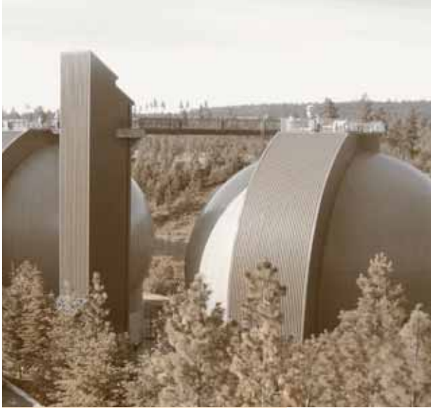
New Digesters at the City's Water Reclamation Plant
