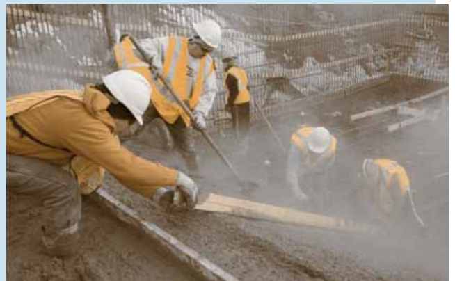
Concrete being poured for the new Shadle Pool.
